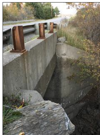
Figure 9 One of four large culverts along the Project area.
