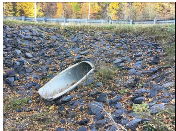
Figure 11 A drainage pipe under US 1.
